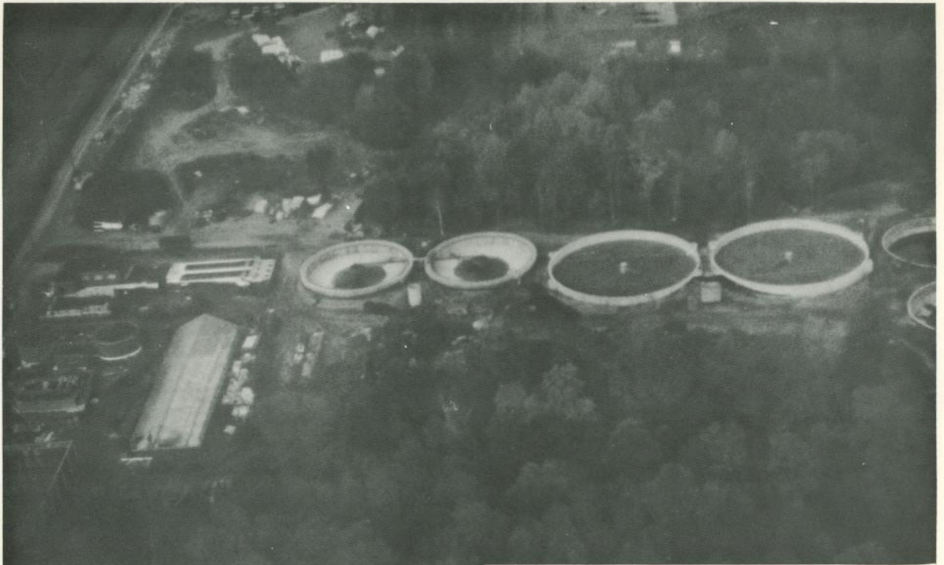
ORANGETOWN SEWAGE TREATMENT PLANT DITMARS AND CARMICHAEL CONSULTING ENGINEERS
